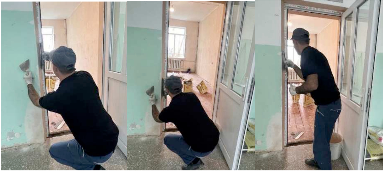
Detailed plastering and smoothing works were carried out on the walls and ceiling.
