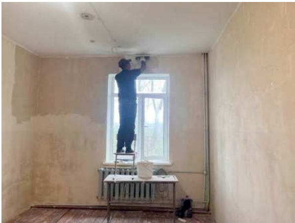
Detailed plastering and smoothing works were carried out on the walls and ceiling.
