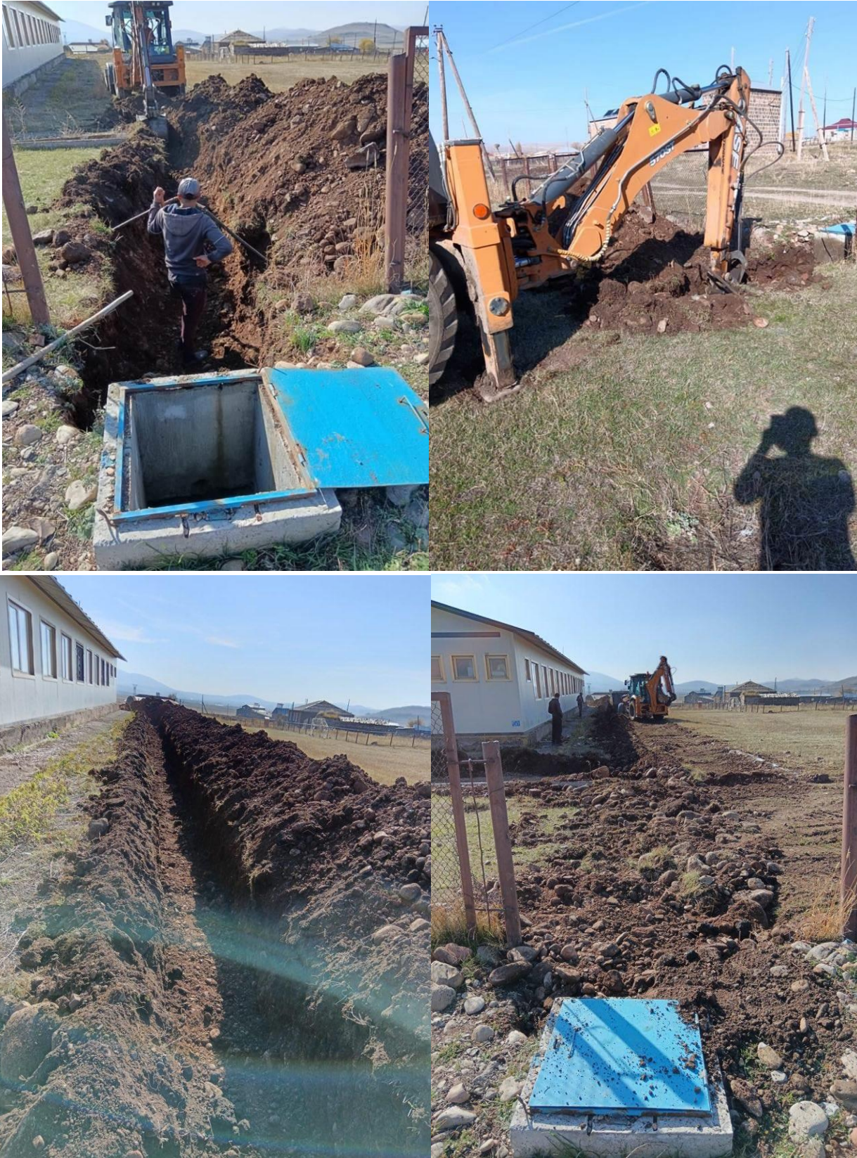
Construction work of new pipeline
